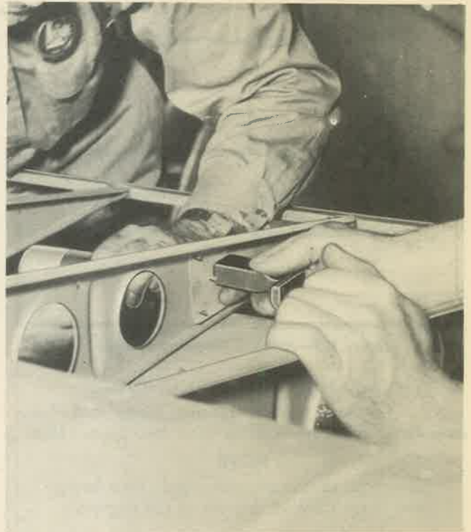
Figure 113—Bucking Rivets—Team Riveting
