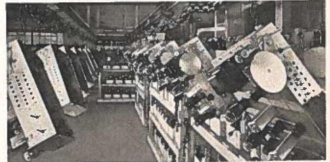
• Assembled chassis move along the conveyor line to final assembly in beautiful Farnsworth cabinets.
