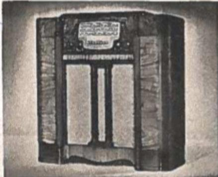
LOW-BOY CONSOLE MODEL AC-91: Period decoration with a modern interpretation. 10 tubes, 5 wave bands, shielded rotatable built-in loop antenna, push-button tuning, 12-inch electro-dynamic speaker, phonograph jack and TELEVISION BRIDGE.
