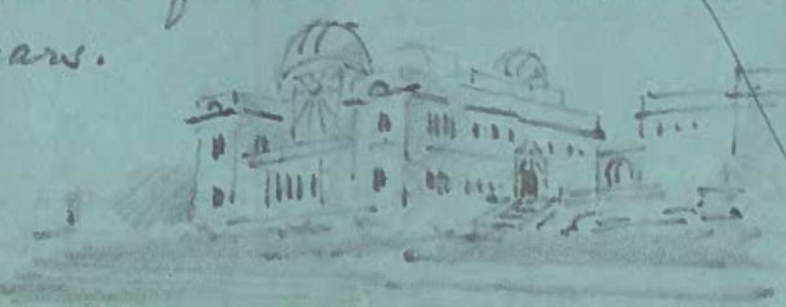
CALIFORNIA ST Looking north west
