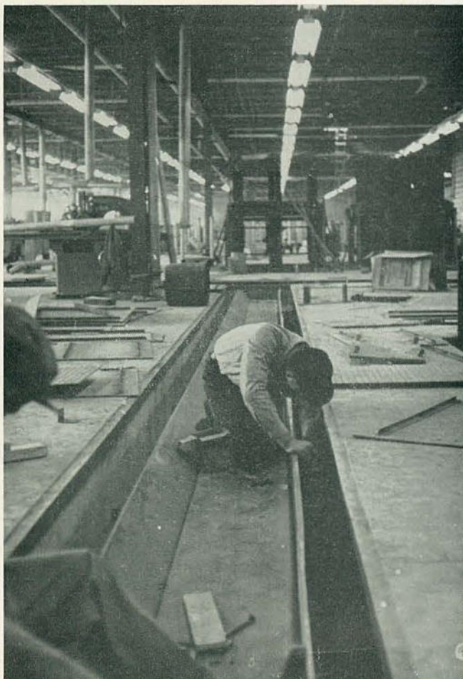
UNDERGROUND CONVEYOR BELTS REMOVE MILL WASTE TO BOILER STORAGE BIN.
